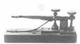
Key-type Morse telegraph transmitter.
